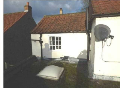
General view of existing first floor bathroom window and flat roof.
